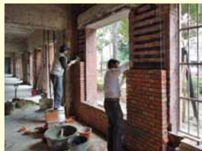
用蔡合源冷凍廠回收 TR 磚新砌圓拱 (f)
