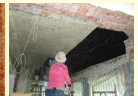
(f) 碳纖貼覆 EPOXY 塗佈
